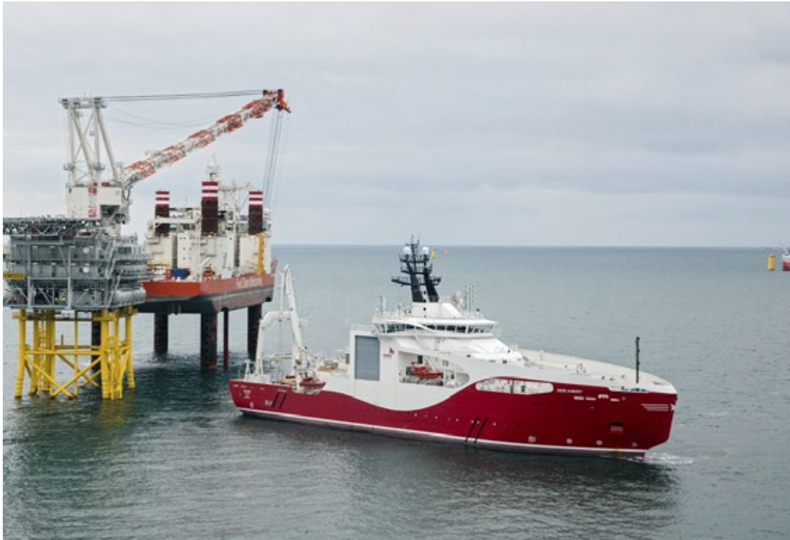
Siem Aimery in action. Photo: Siem Offshore Contractors GmbH
