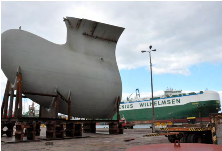
New bow bulb was installed on vehicle carrier *Figaro* at Remontowa SA. Photo: Jerzy Uklejewski
